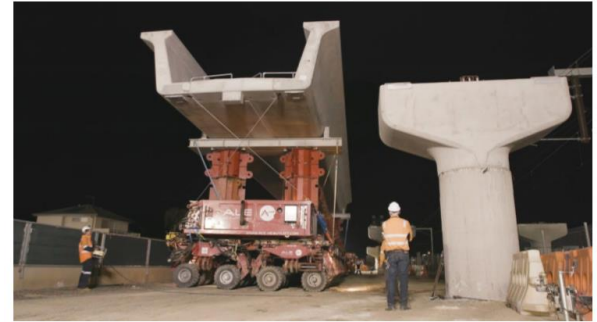
This bridge is strong because of its u shaped deck
